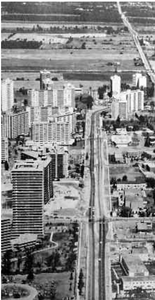
Fig. 8. Bathurst Green Belt: Tower cluster at Metro's Northern border, with untouched farmland beyond
